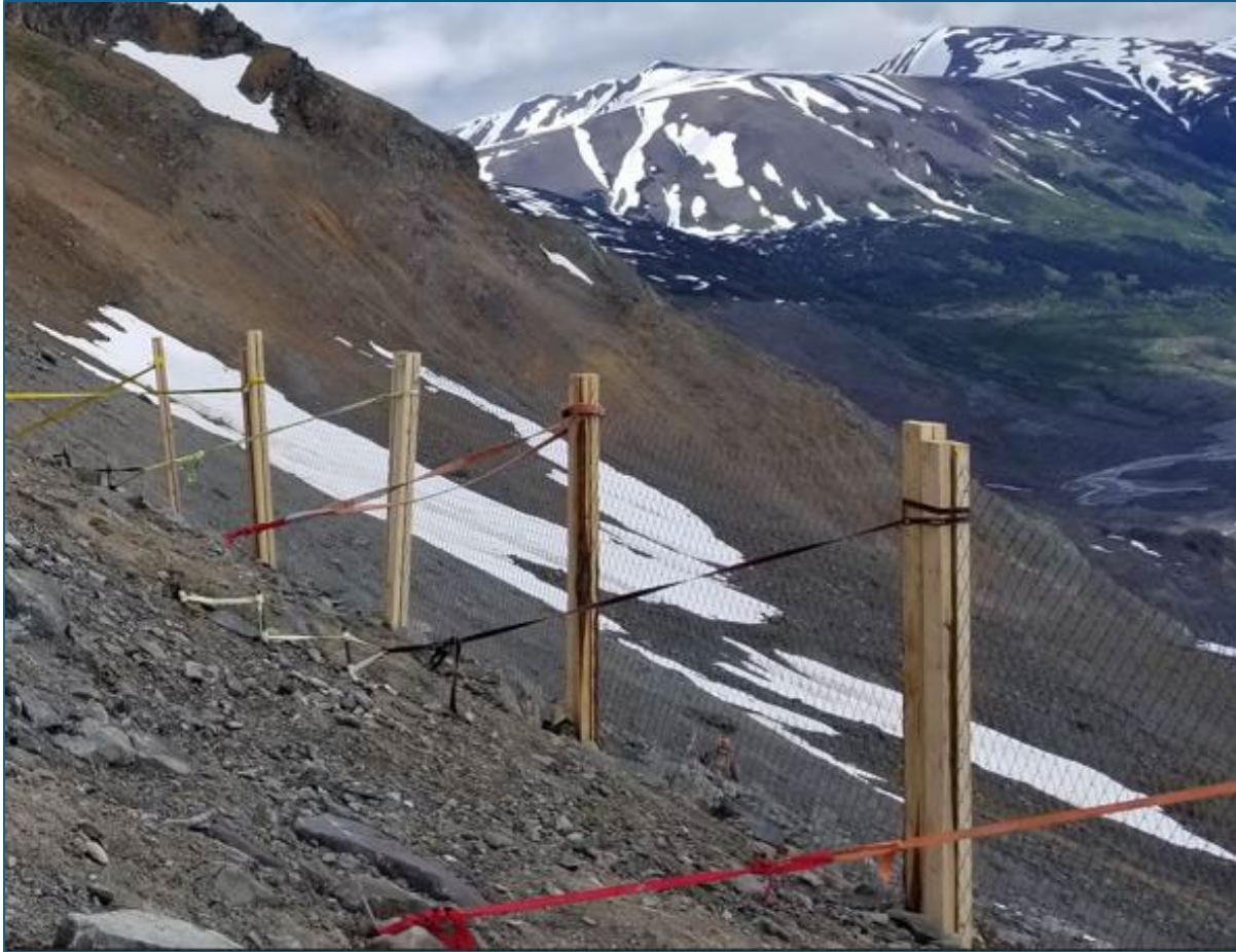
Figure 5. Non-engineered rockfall protection array. Note wooden posts.
