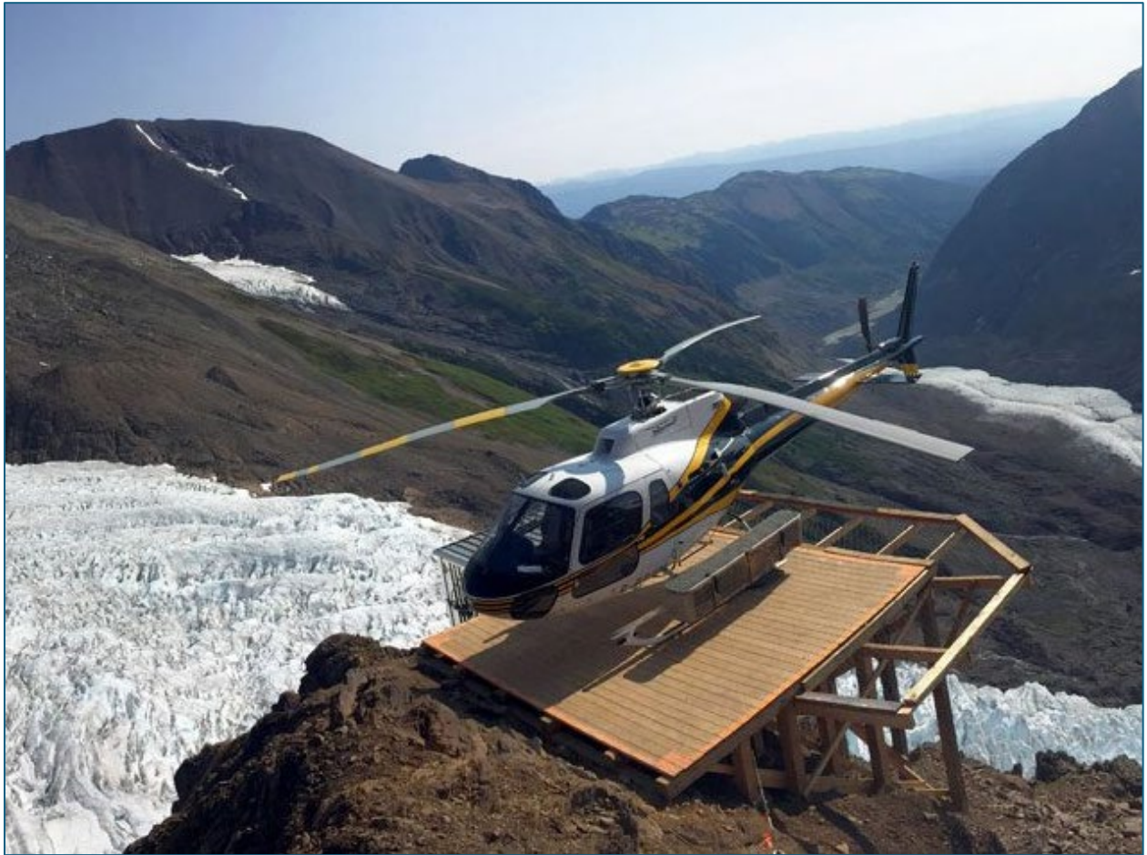
Figure 3. Timber helicopter pad. Each helicopter supported drilling site will have a helicopter pad to facilitate emergency response and exploration operations. Note "aircraft carrier" type fall protection surrounding the pad to prevent falling from height.
